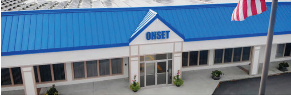
Onset headquarters, Cape Cod, MA
